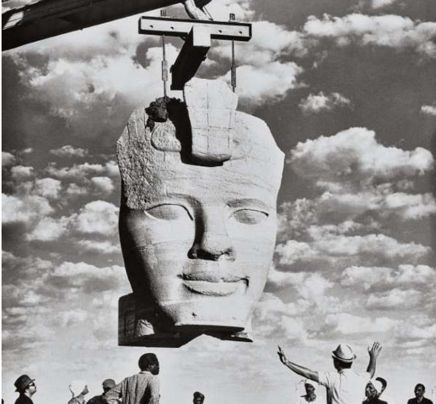
Abu Simbel: One of the most delicate – and spectacular - tasks: the face of Ramesses II is accurately moved. It is almost ready to be repositioned on the pharaoh's statue (1966)
